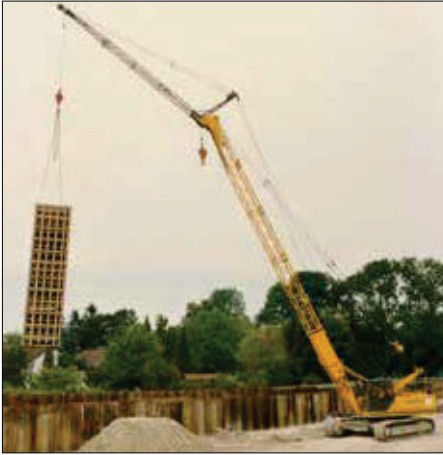
1976-1995: S 1225 crawler crane with fly boom to lift casing boards
